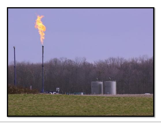
Above: Typical site for oil production without gas capture. Oil and water are collected in the tanks and the gas is released through a flare stack or vented to the atmosphere.
