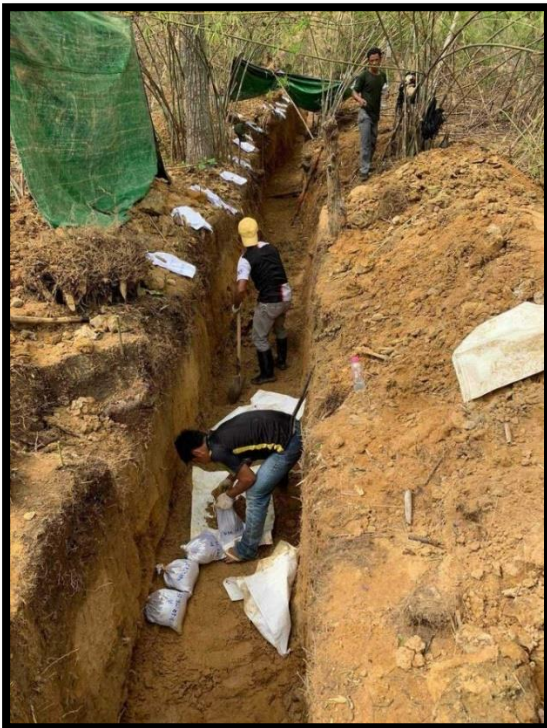
Figure 1 left Trenching and Sampling at Wild Boar
