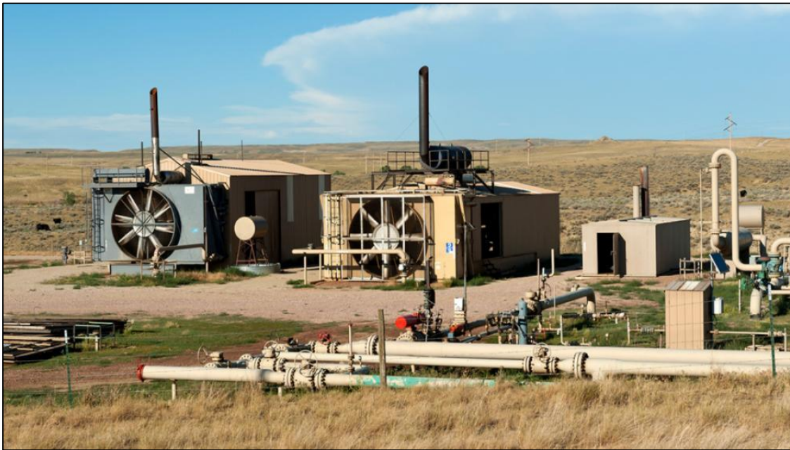
Typical dual compression processing site connected via pipeline to oil production sites.
