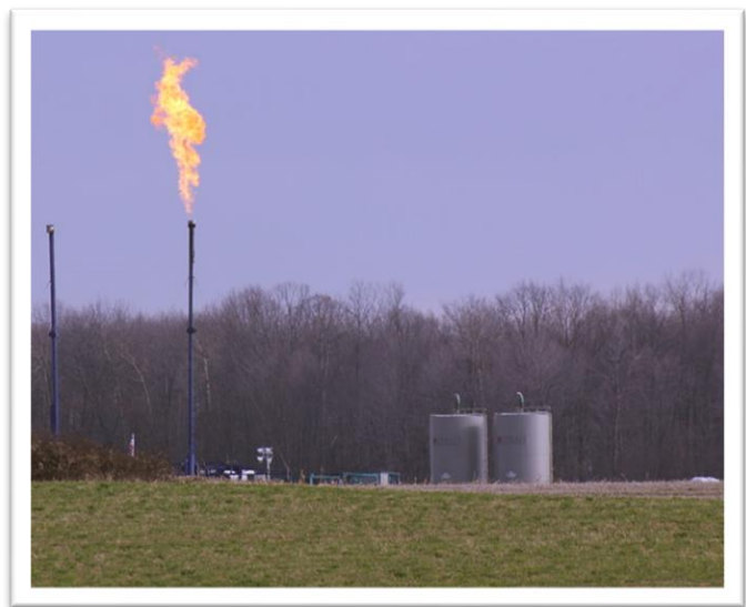
Examples of oil storage tanks venting and flaring.
