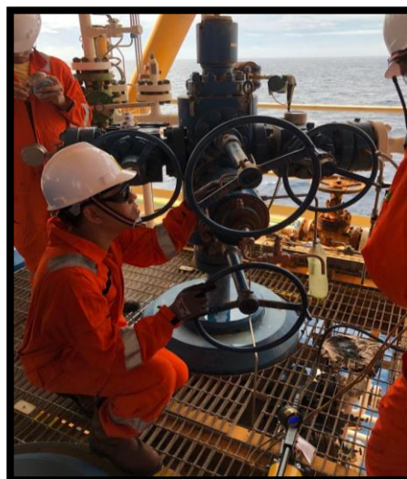
Figure 2: Technicians take pressures during inspection.
