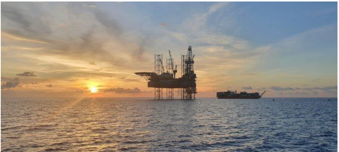
Offshore drilling platform with production barge nearby.
