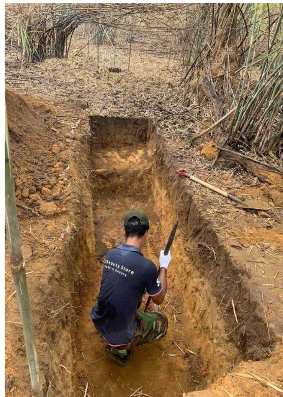
Angkor staff complete shallow trenches following multiple gold-bearing veins identified during its recent pitting program. Veins will be mapped, sampled and assayed for grade, intersections, thickness, and dip or strike.
